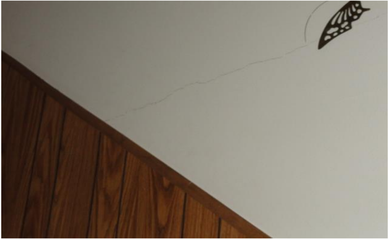
Photo # 12 Crack between beams, left side of ceiling in family room
