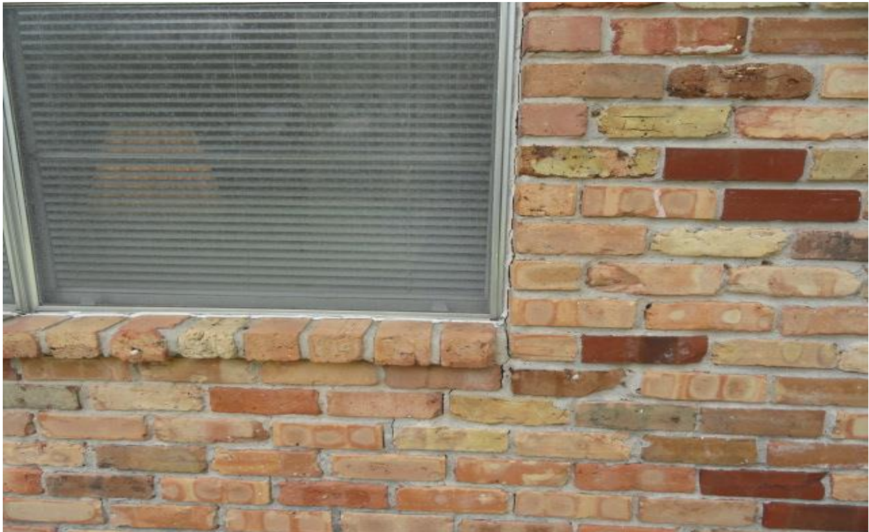
Photo # 6 Crack at bottom left of family room window, with caulk separation at brick
