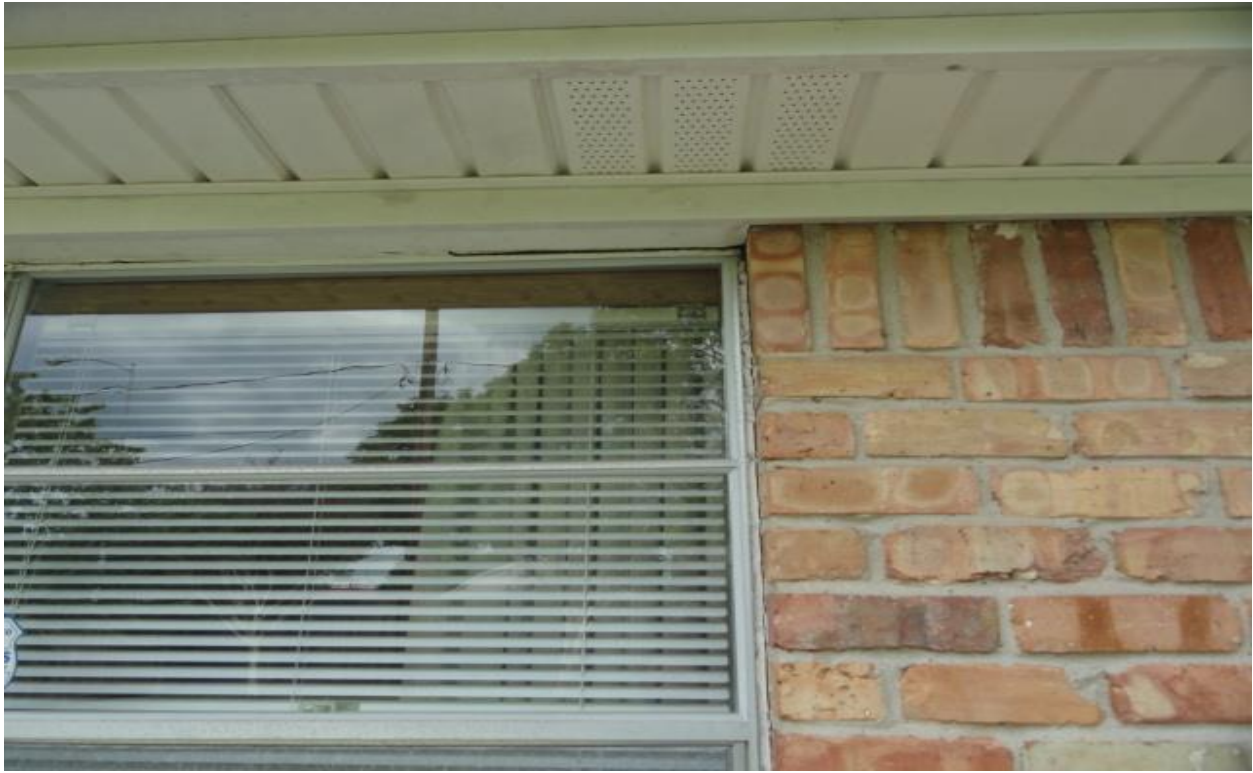
Photo # 8 Separation of top trim at top of window
