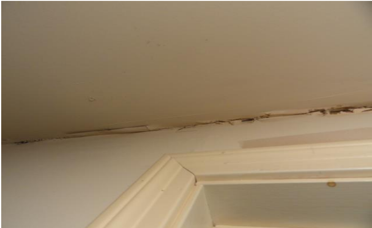
Photo # 24 Cracking along ceiling/wall in front closet of upstairs left bedroom
