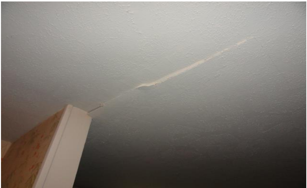
Photo # 20 Fallen sheetrock in living room ceiling at foyer
