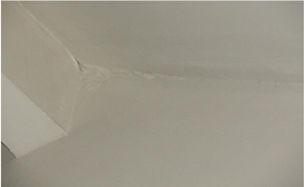
Photo # 14 Cracks in front wall under second floor landing, at floor/wall transition
