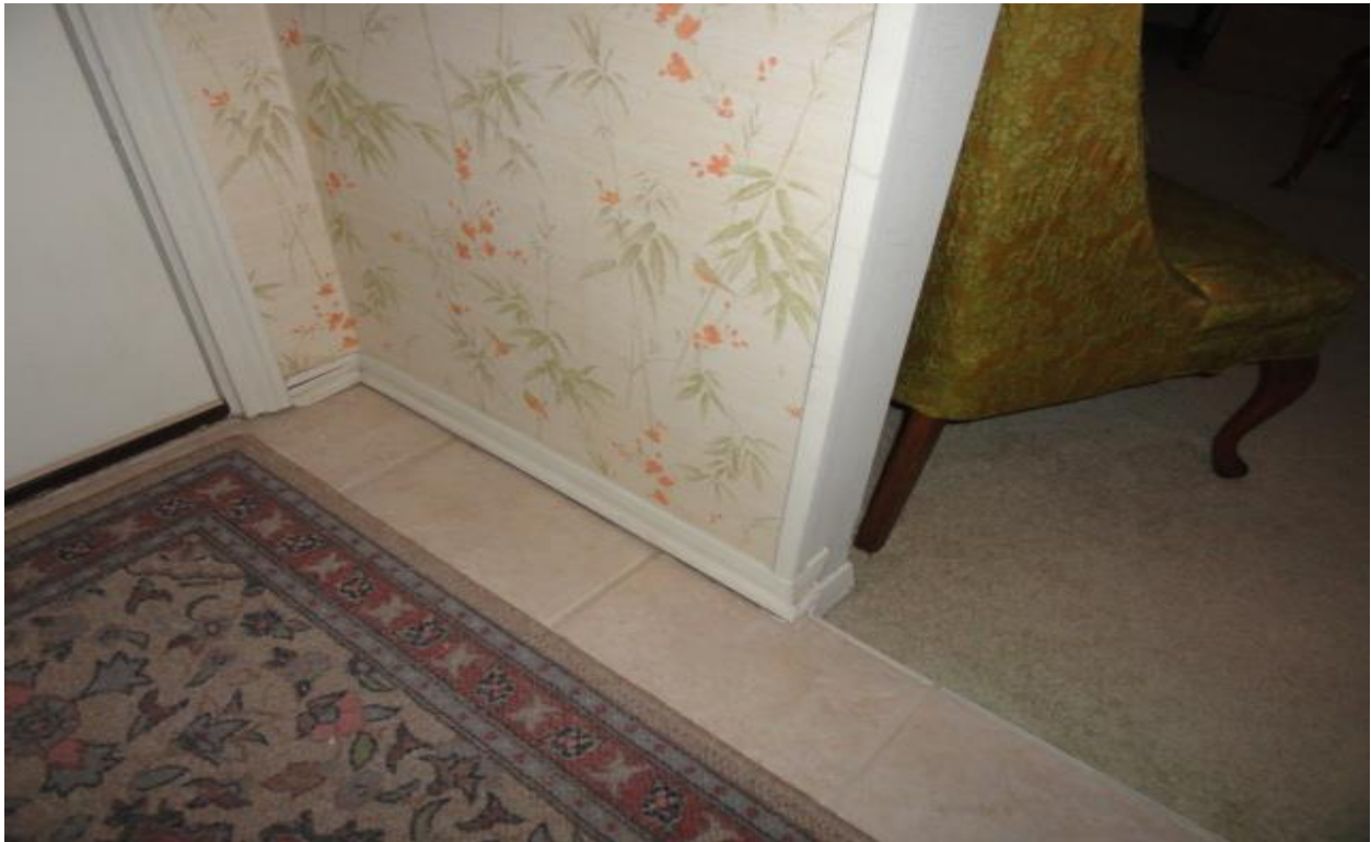
Photo # 22 Separation of wall at left front of foyer from floor
