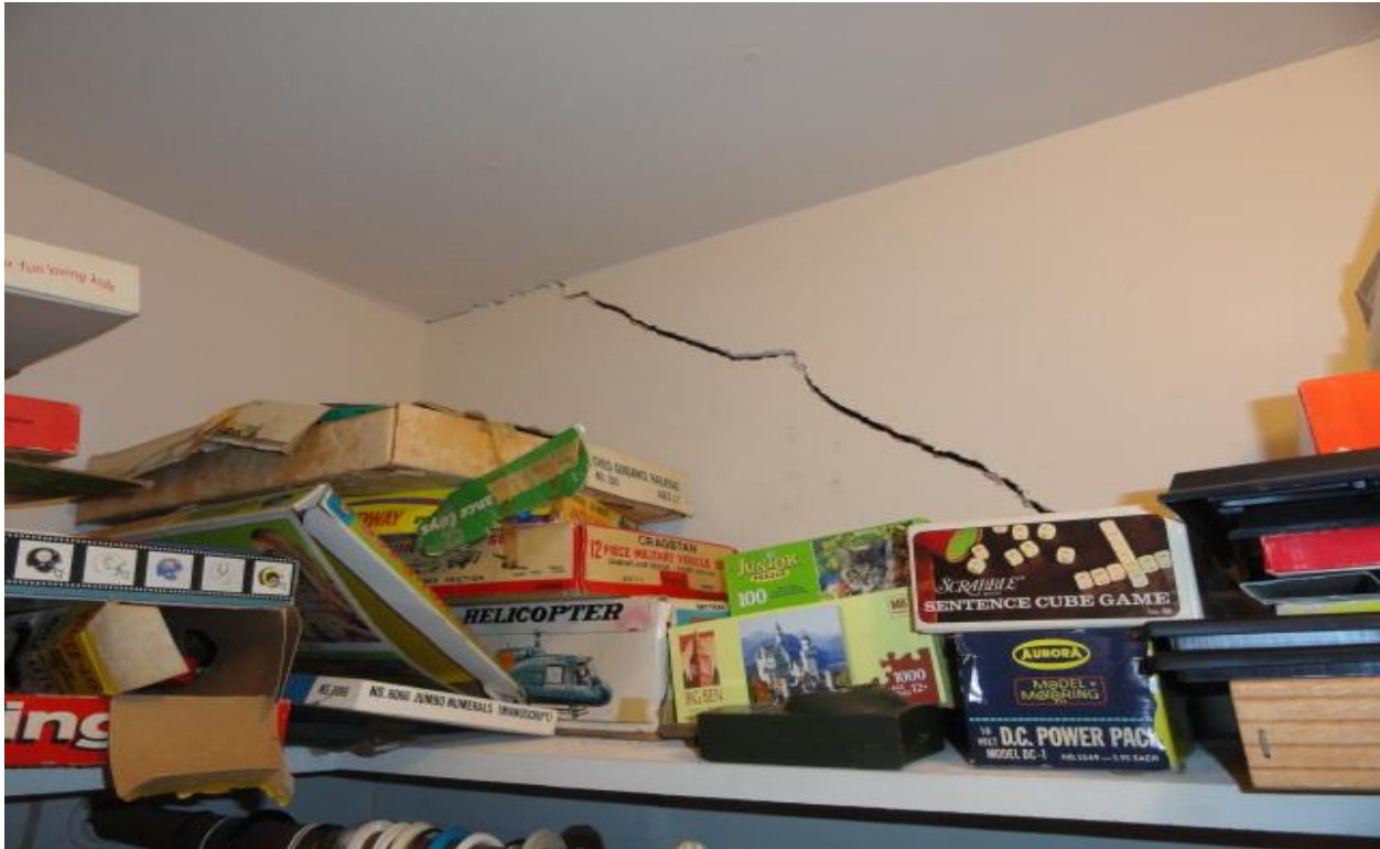
Photo # 24 Cracking along ceiling/wall in front closet of upstairs left bedroom
