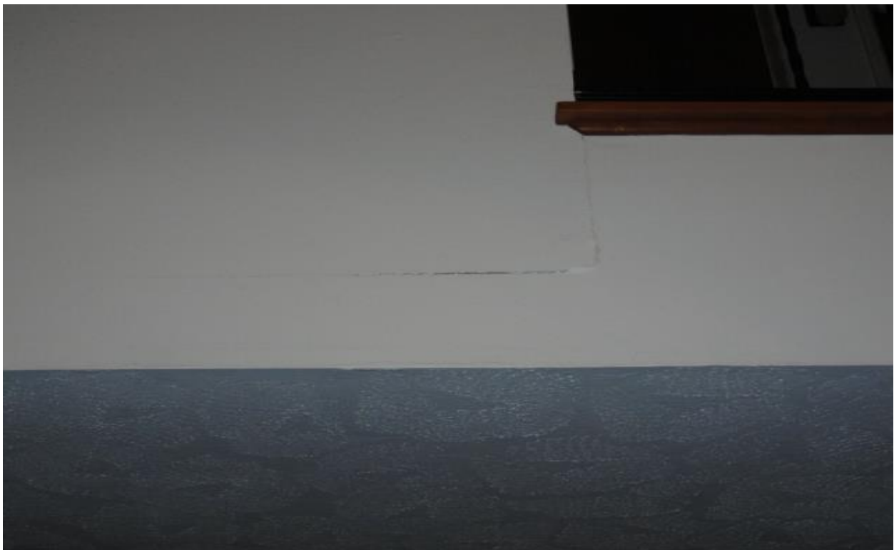
Photo # 14 Cracks in front wall under second floor landing, at floor/wall transition
