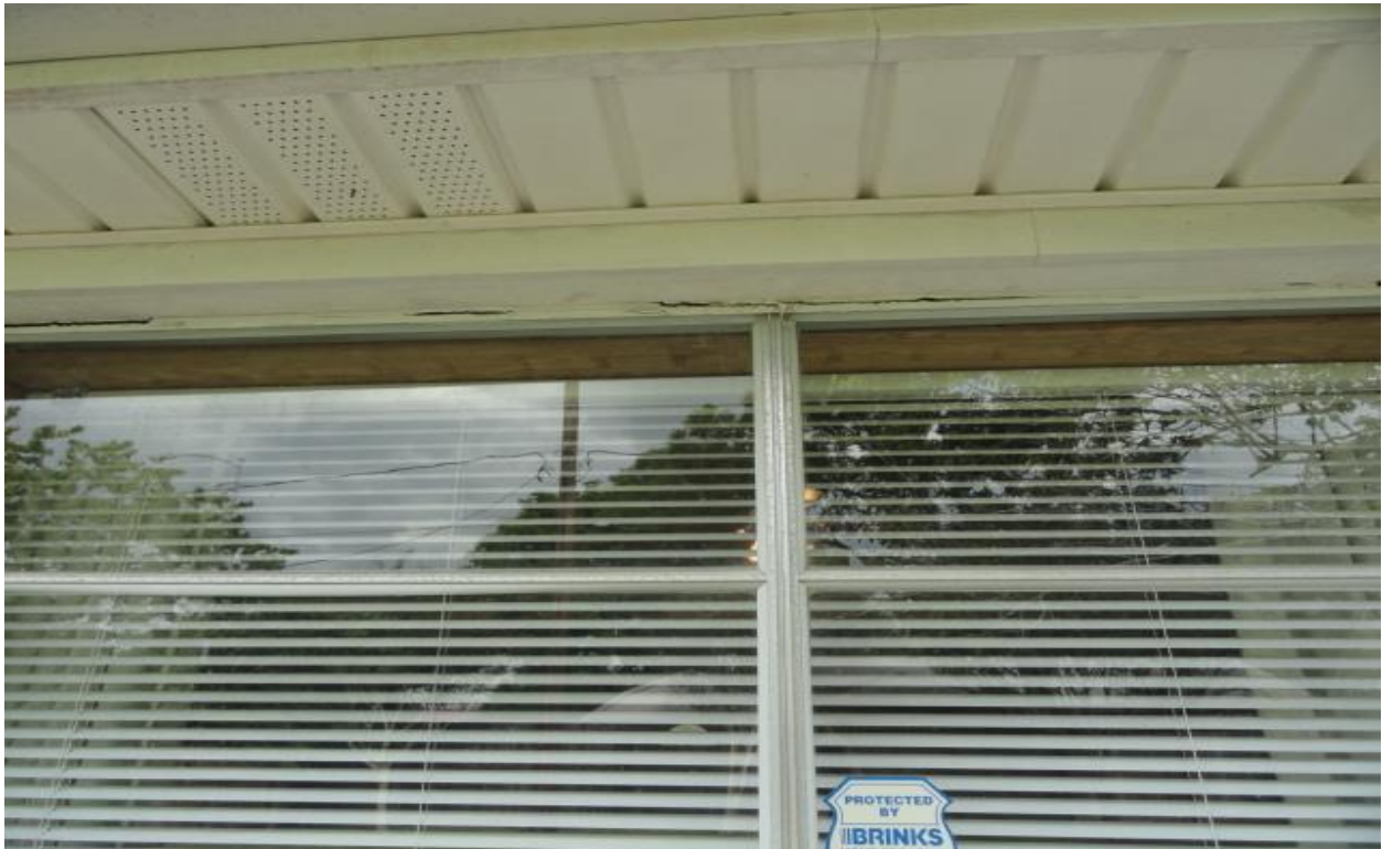
Photo # 8 Separation of top trim at top of window
