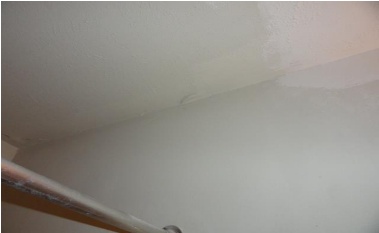
Photo # 16 Cracking and repair at wall/ceiling over bathtub
