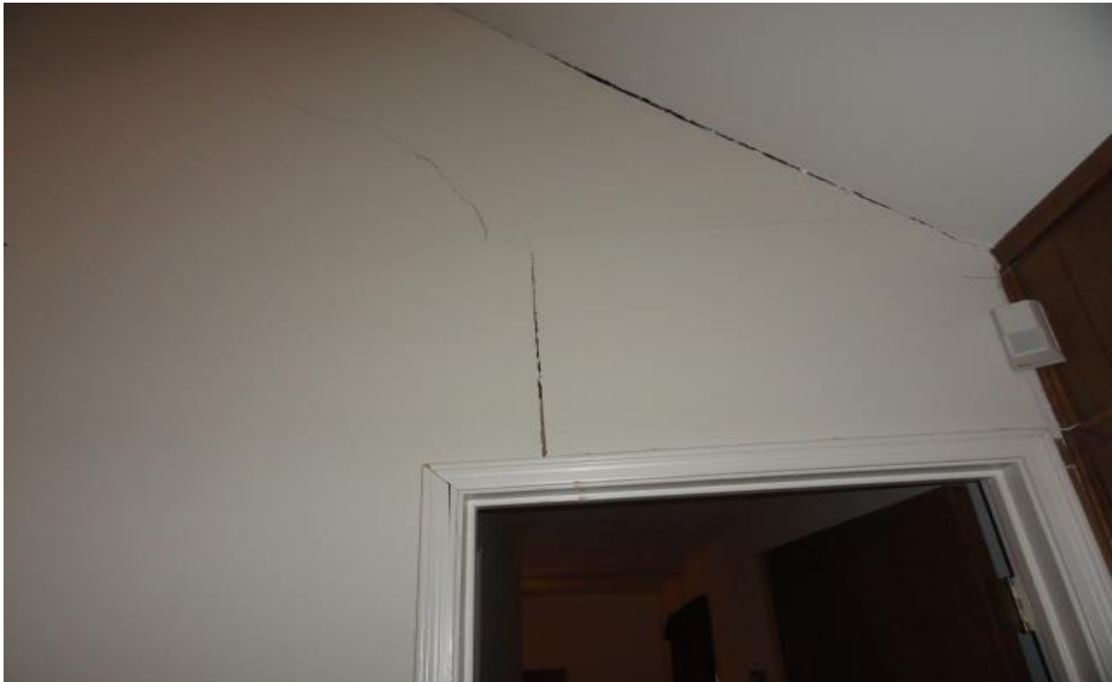
Photo # 10 Cracks above door to master bedroom
