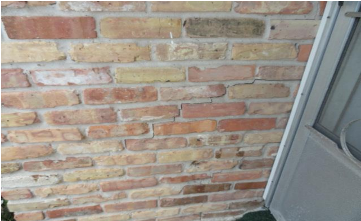
Photo # 2 Cracks in brick to left of front entry door
