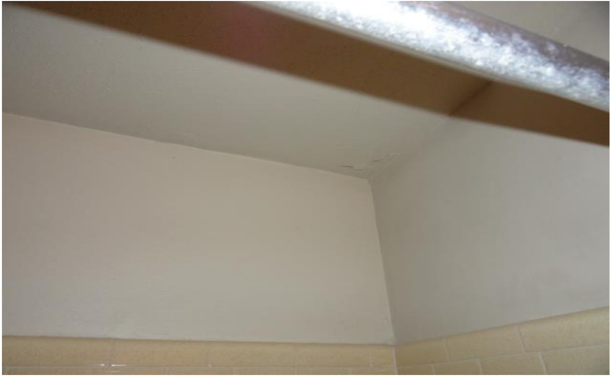
Photo # 16 Cracking and repair at wall/ceiling over bathtub
