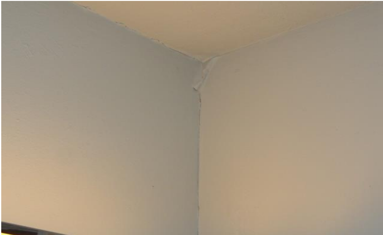
Photo # 18 Sheetrock damage in master bedroom
