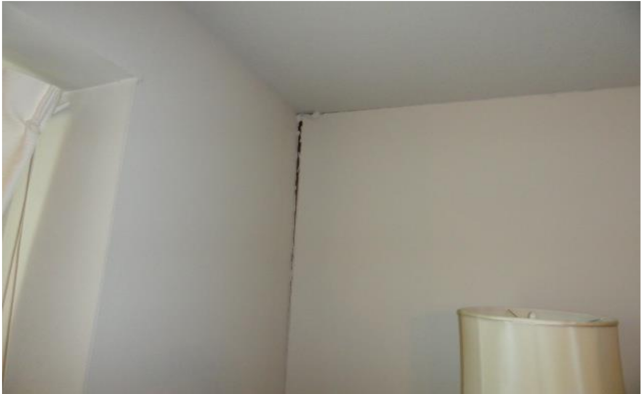
Photo # 22 Separation of wall at left front of foyer from floor
